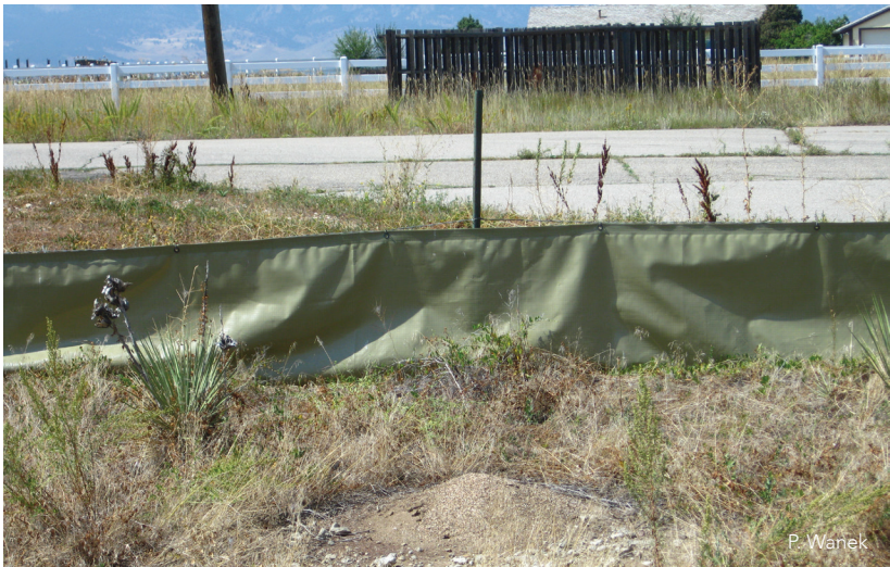
Flawed vinyl barrier installation.
