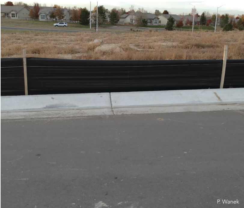
Silt fence with stakes and staples exposed.
