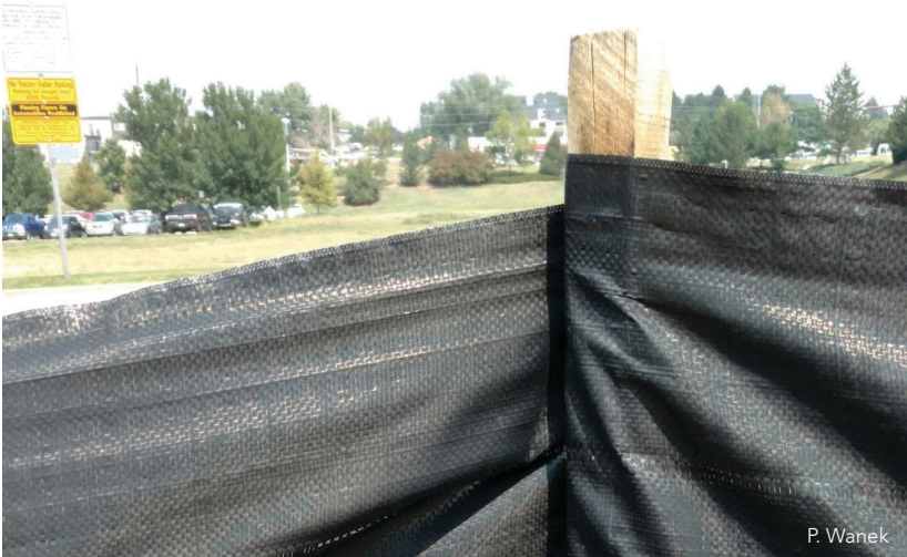
Modification: Twist fabric around stake for longevity.
