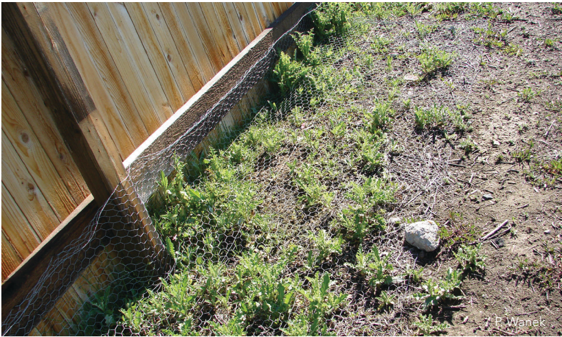
B. Skirting attached to prairie dog side of fence.
