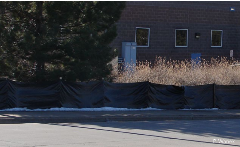
Silt fence used for pending construction.
