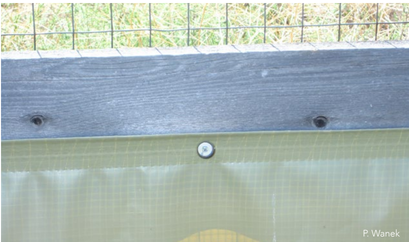
Screw and washer through grommet
