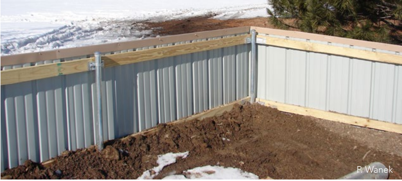
Prairie dog side of barrier. Note wildlife safe caps on metal posts and elongated cap along top of metal fencing.
