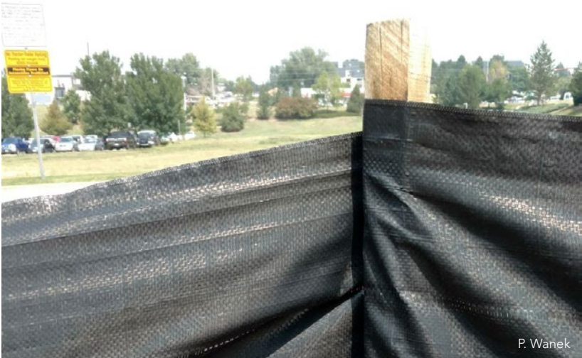
Modification: Twist fabric around stake for longevity.
