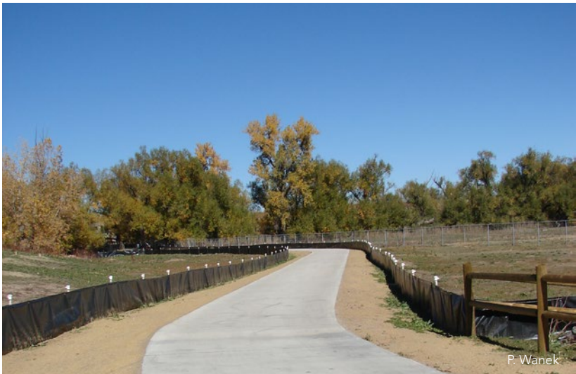
Temporary vinyl barrier used during construction project.
