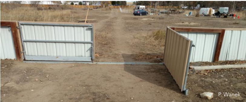
Gates for vehicle access. Culvert pipe at threshold blocks light.
