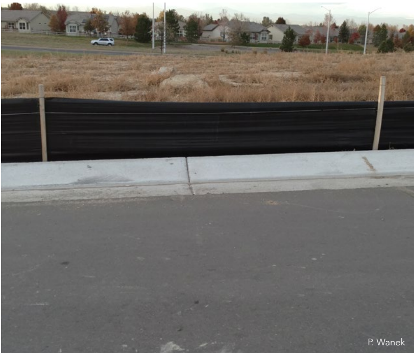
Silt fence with stakes and staples exposed.
