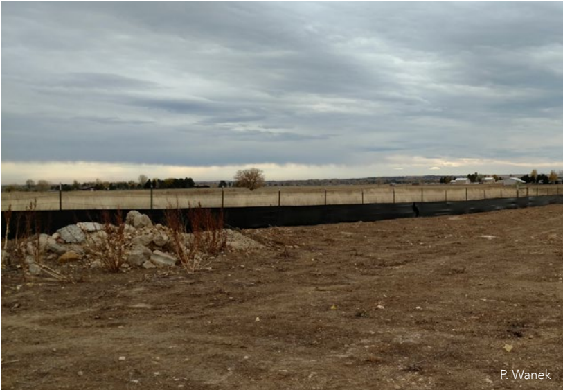
Silt fence used in large field.
