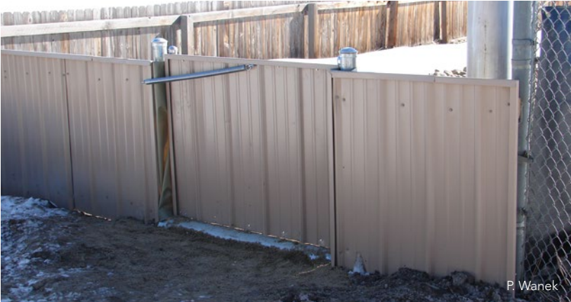
Self-closing swing gate for pedestrians (springs on each side of gate). Metal culvert pipe at threshold blocks light.
