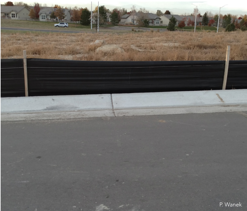
Silt fence with stakes and staples exposed.
