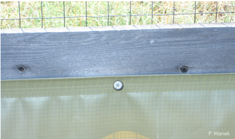
Screw and washer through grommet
