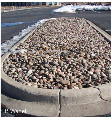
Parking lot median
