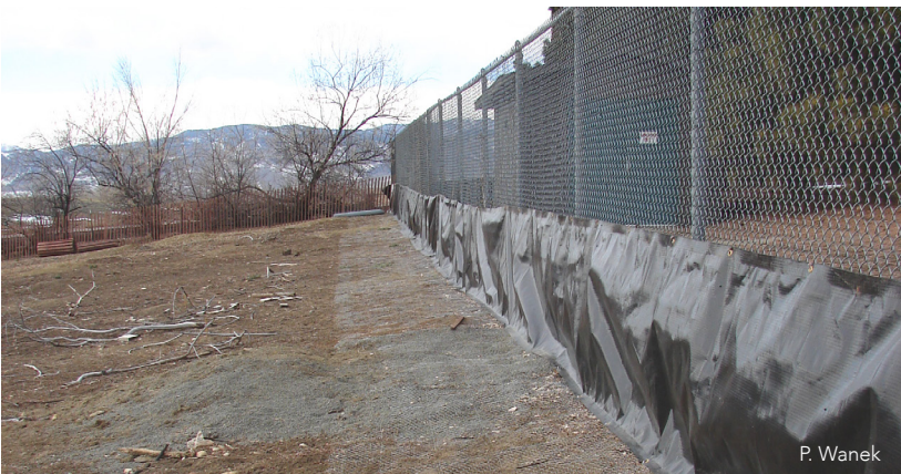
Modified existing chain-link fence to inhibit movement back into park. (prairie dog side)
