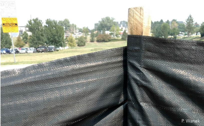
Modification: Twist fabric around stake for longevity.
