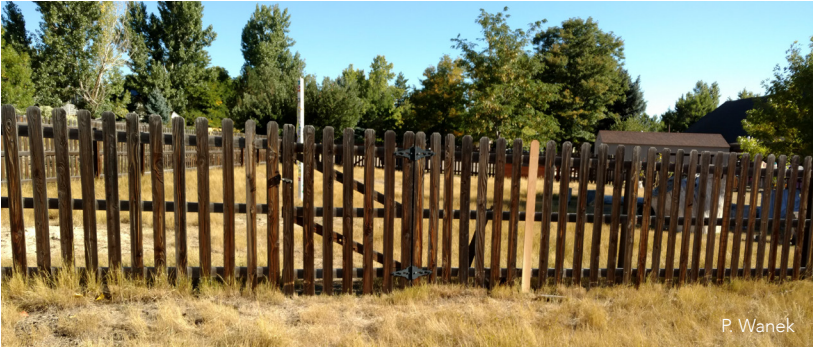
A. Existing fence before modifications.
