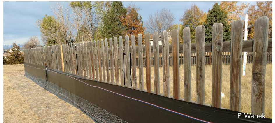
B. Modified to exclude prairie dogs by adding black silt fence and skirting.
