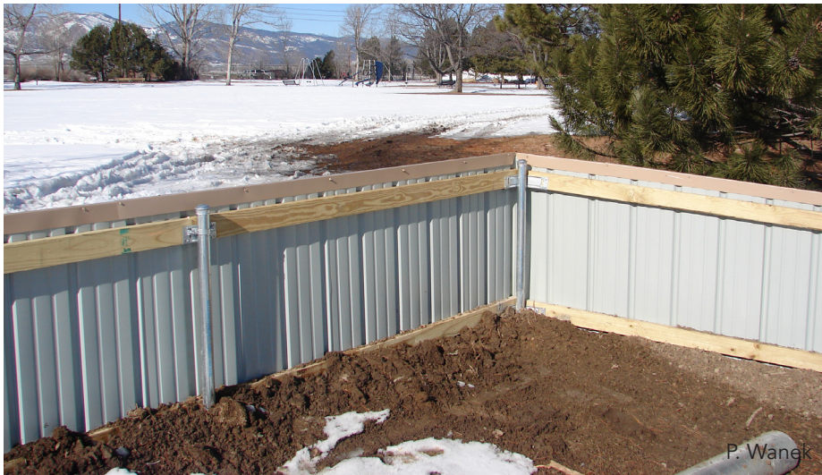
Prairie dog side of barrier. Note wildlife safe caps on metal posts and elongated cap along top of metal fencing.
