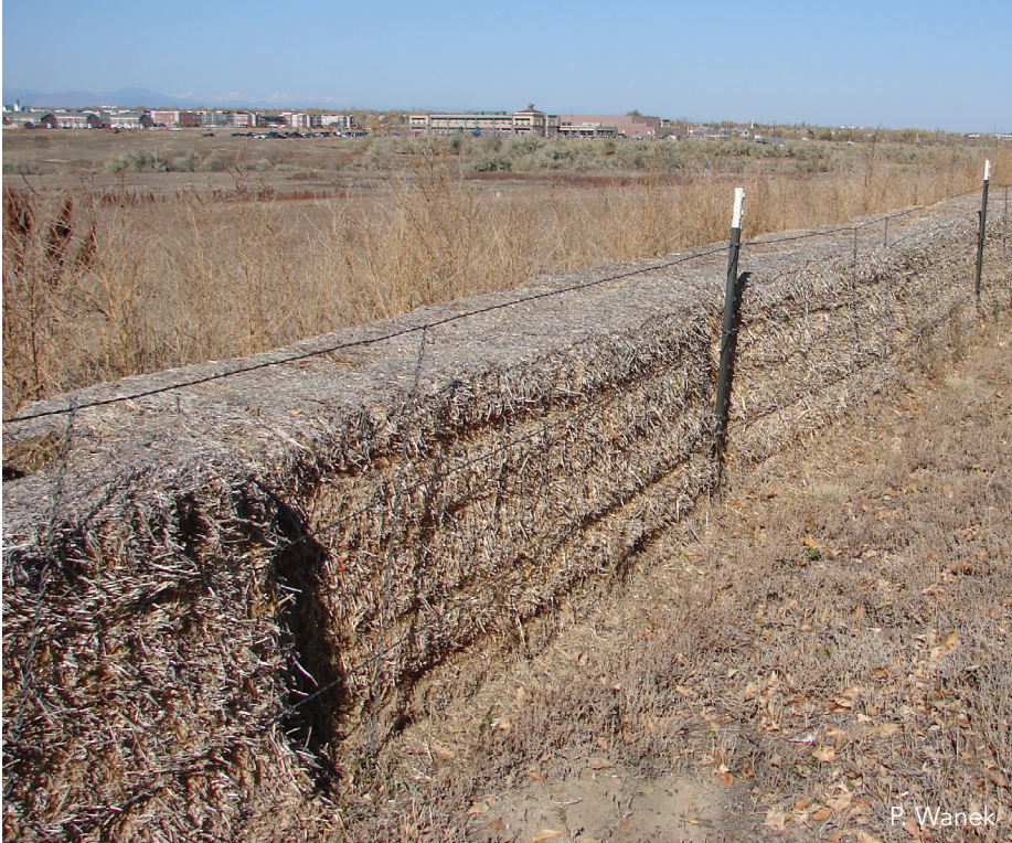
Straw bales along prairie dog side of fencing.
