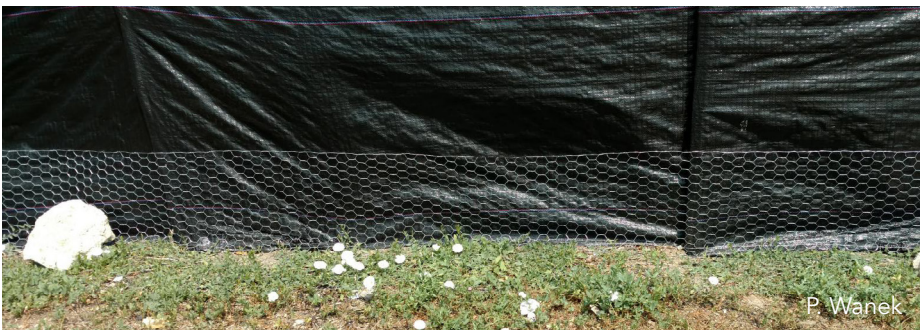
Modification: Using two-foot wide one-inch netting poultry wire, lip one foot vertically and use a staple gun to attach to wood posts. Anchor horizontal piece to ground with six-inch pins.
