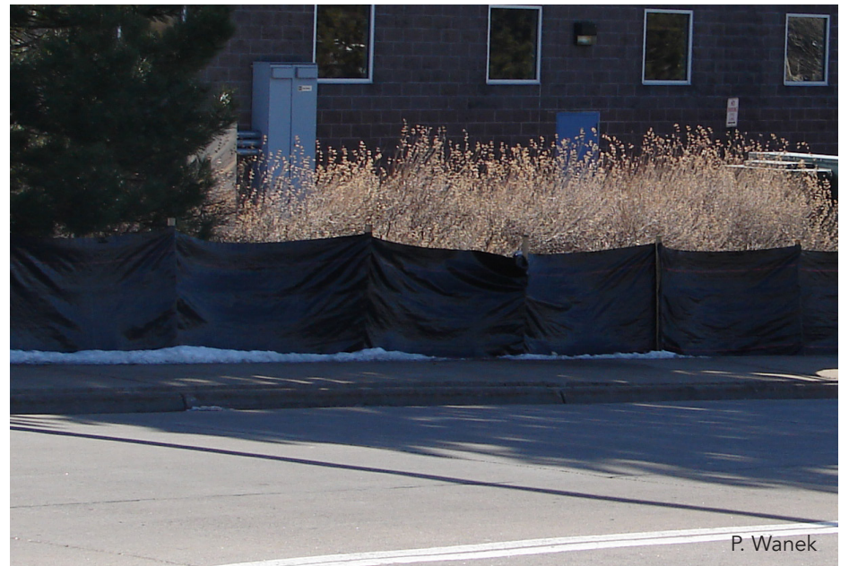
Silt fence used for pending construction.
