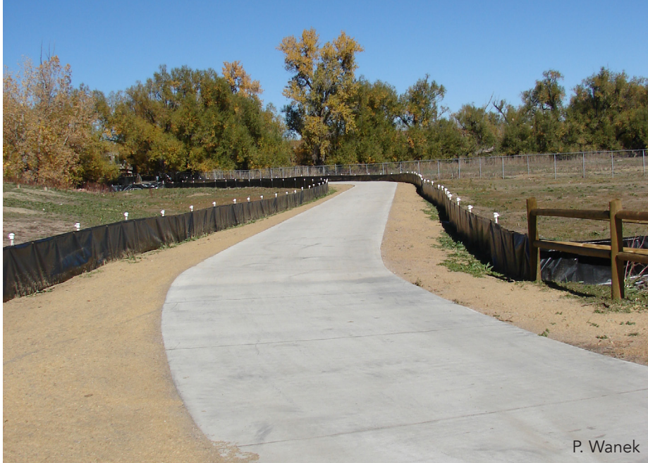
Temporary vinyl barrier used during construction project.
