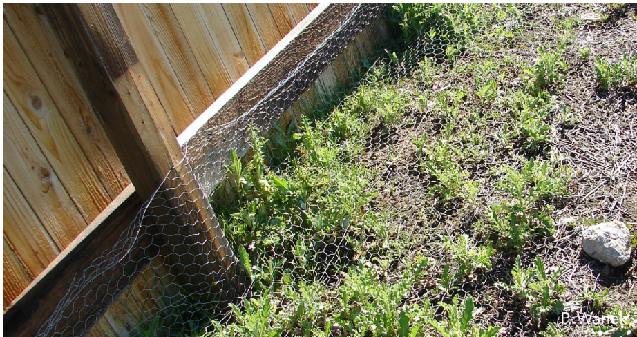
B. Skirting attached to prairie dog side of fence.
