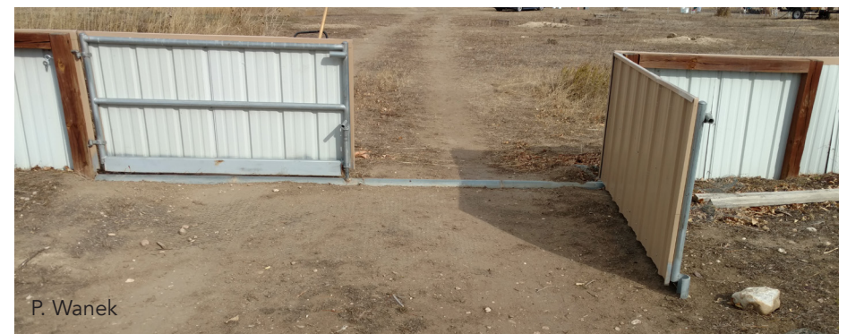
Gates for vehicle access. Culvert pipe at threshold blocks light.
