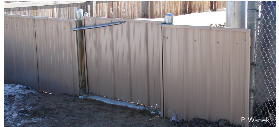
Self-closing swing gate for pedestrians (springs on each side of gate). Metal culvert pipe at threshold blocks light.
