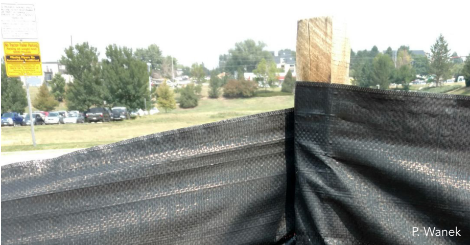
Modification: Twist fabric around stake for longevity.
