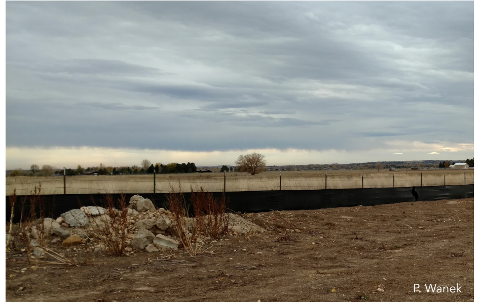
Silt fence used in large field.
