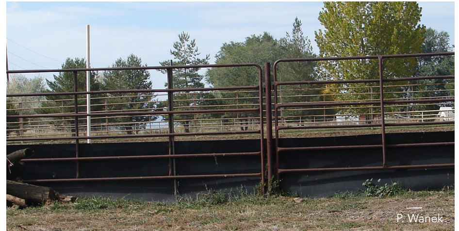
Example #1 - Recycled mining conveyor belts – used against a horse arena provides a good visual and physical deterrent. Arena kick boards could also be effective.
